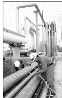
CONAM's PCMS group pinpoints erosion and corrosion with the help of the program.
